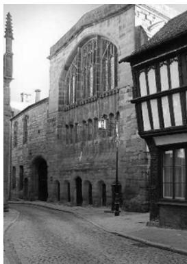
Part of the old City of Coventry incl' Church of St Marys
